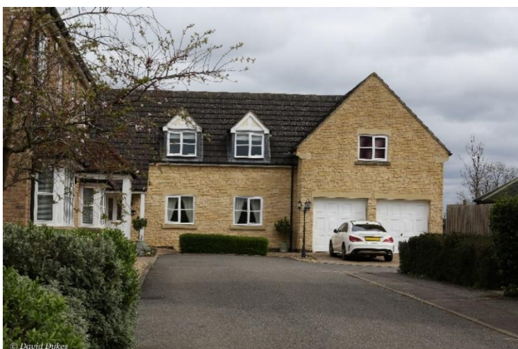
Picture 7: Eastwell Court, another small development demonstrating use of traditional materials.
